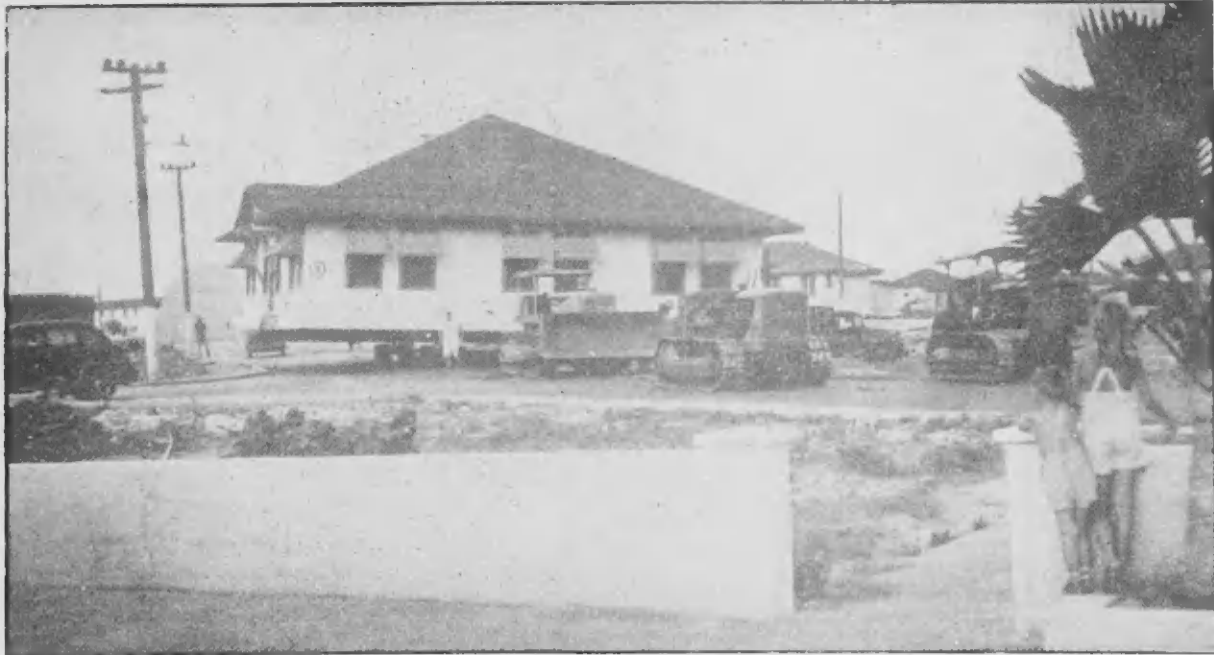
Lago's second biggest moving job (the biggest was when the Hospital was moved ten years ago) occurred June 27 when the Utilities office was hoisted up on dollies and moved from its old location north of the Instrument Shop to its new site next to Powerhouse No. 2. The house is shown above temporarily blocking the road just below the Colony Post Office. The figure in the white shorts is John Pfaff, of the Transportation Dept., who stopped off for a moment to see how things were going.
